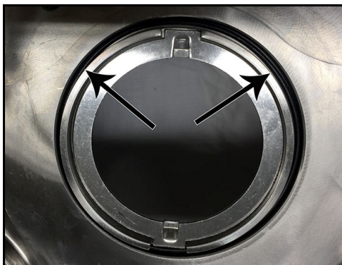
Figure 89 - Seal housing O-ring installed
